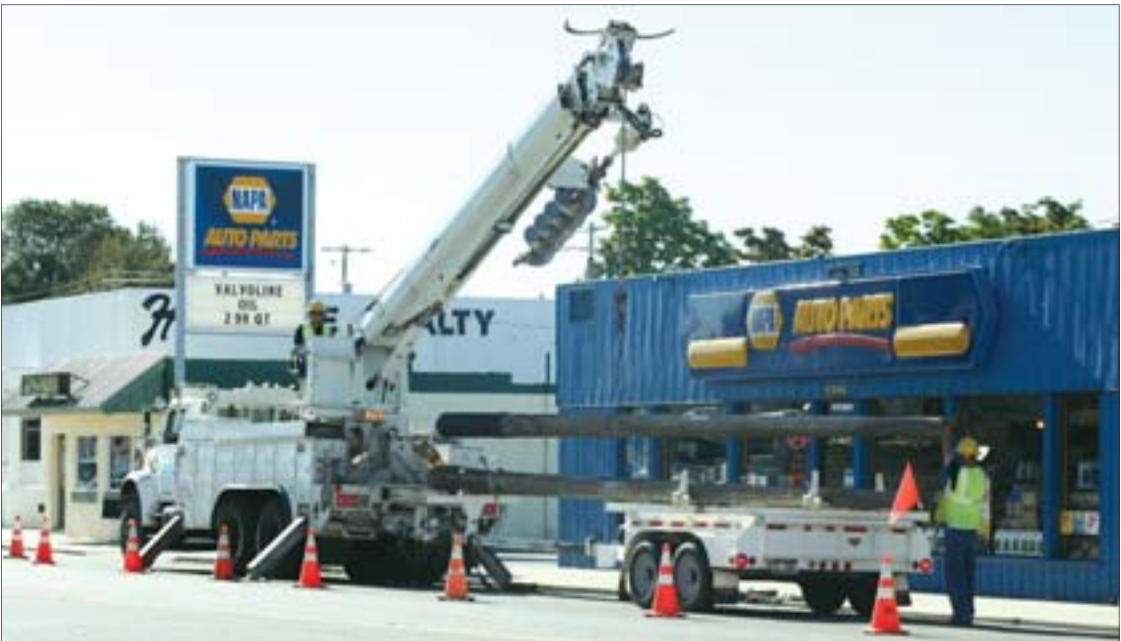
Idaho Power crew removes an old light pole from in front of NAPA Auto Parts on East Idaho Avenue in Homedale on Wednesday. The work was part of removal of nearly every wooden power pole along the street as part of the Local Improvement District revitalization project.
